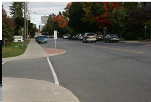
The Figure above shows a curb extension on Holland Avenue in an area of on-street parking. (McCormick Rankin Corporation). The Figure at left is an example of how a curb extension helps to make a pedestrian more visible by locating the refuge area closer to the travel lane. ([www.pedbikeimages.org/](http://www.pedbikeimages.org/) Dan Burden)
