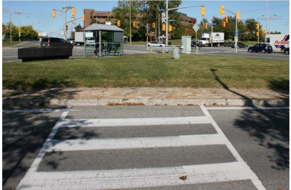
In this photo, a crosswalk is provided across a channelized right turn lane at the Baseline / Prince of Wales intersection. At this location there is no curb ramp, a very rough texturized sidewalk treatment not conducive to mobility challenged or pedestrians requiring assistive devices, and a very limited refuge area. These types of conditions present significant challenges for pedestrians. (McCormick Rankin Corporation)
