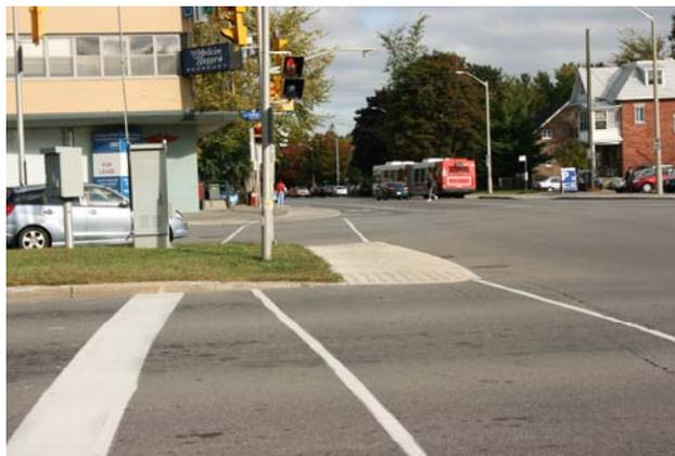
Median refuge islands allow pedestrians to focus on crossing one direction of traffic at a time and provide a refuge area to wait for a gap in traffic partway through the crossing. There must, however, be space to accommodate the volume and mix of pedestrians using the crossing (i.e. wheelchairs, strollers, etc.). (McCormick Rankin Corporation)
