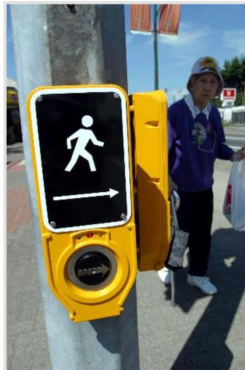
The above APS push-button is one example of the many types that provide a locator tone to help visually impaired pedestrians find it and provides audio and vibrotactile feedback corresponding to the "walk" indication in the crossing direction indicated by the tactile arrow. ([www.pedbikeimages.org](http://www.pedbikeimages.org/) / Dan Burden)
