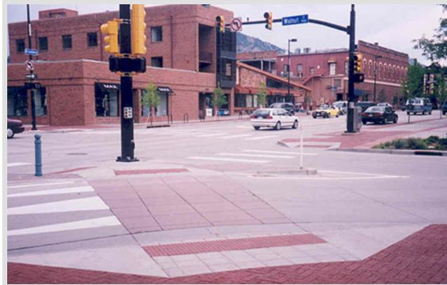
In this photo, a raised crosswalk is placed across a channelized slip lane to help reduce vehicle speeds and improve awareness of pedestrians. Note the texturized pavement and curb ramp that help transition from the sidewalk to the crosswalk. ([www.pedbikeimages.org](http://www.pedbikeimages.org) / Dan Burden)
