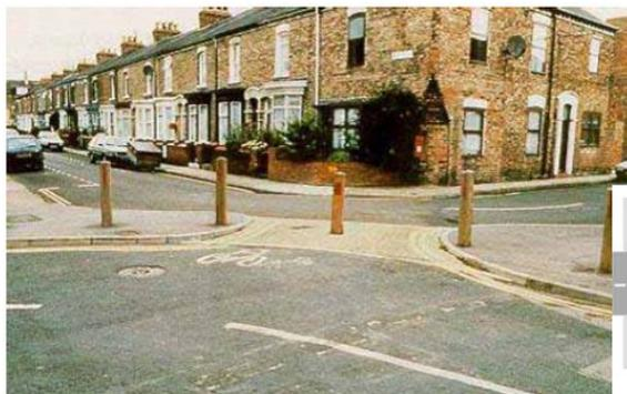
The above photo illustrates a diagonal diverter with removable bollards for emergency access. To the right are examples of the four basic types of traffic diverters. (FHWA University Course on Bicycle and Pedestrian Transportation)
