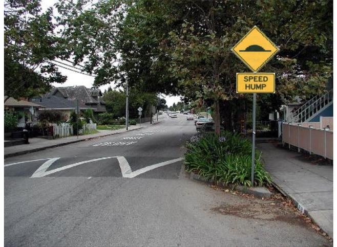
Speed humps and tables are often used to help reduce vehicle speeds in advance of pedestrian crossing areas. (Dan Burden / McCormick Rankin)
