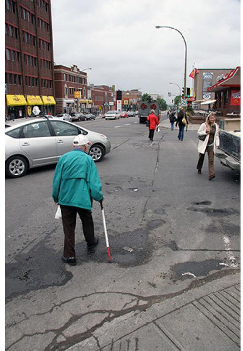
In the above photo, the deteriorated pavement markings make it difficult for drivers to detect its presence. (www.pedbikeimages.org / Dan Burden)
