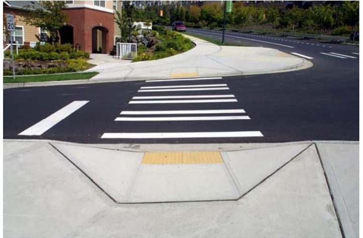
An example of a curb ramp to provide an adequate transition between the sidewalk and roadway. This particular installation has a texturized and coloured pad at the bottom of the ramp to assist special needs pedestrians but its use is not standard practice in Ottawa. ([www.pedbikeimages.org](http://www.pedbikeimages.org/) / Dan Burden)
