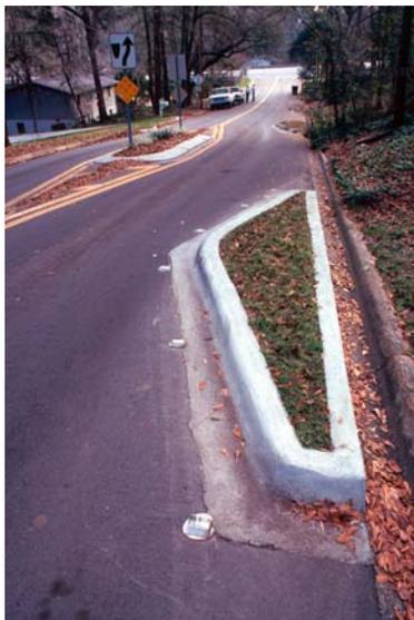
The photos above and at right provide examples of a chicane located between intersections. They require a vehicle to shift laterally and if designed properly will reduce operating speeds. ([www.pedbikeimages.com](http://www.pedbikeimages.com/) / Dan Burden)
