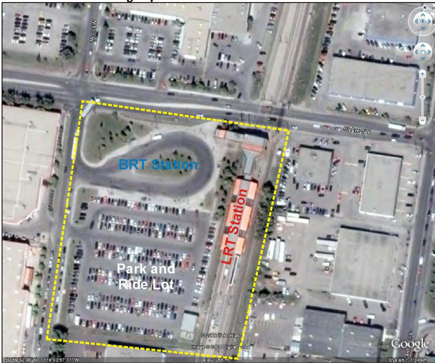
Calgary 61st Street Transfer Station
