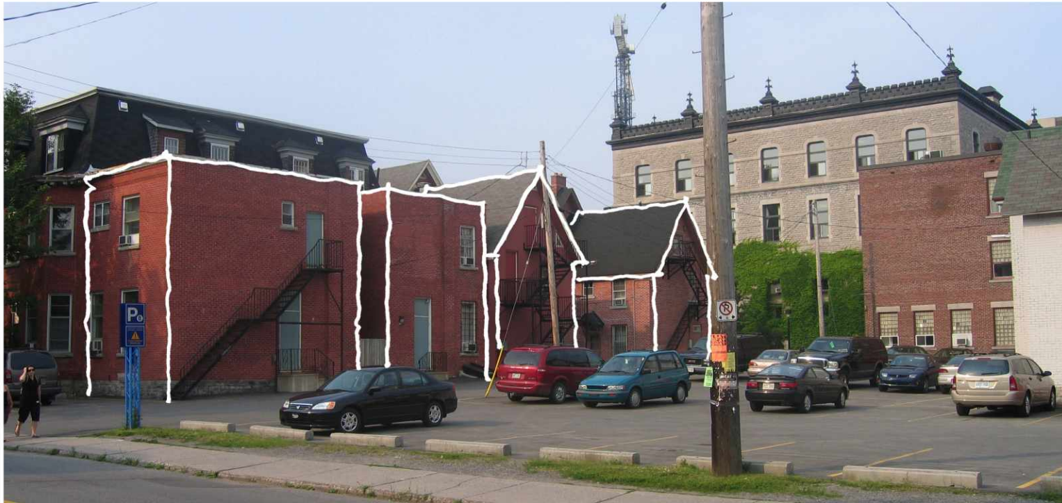
VIEW FROM CUMBERLAND STREET SHOWING REAR ADDITIONS TO BE DEMOLISHED
