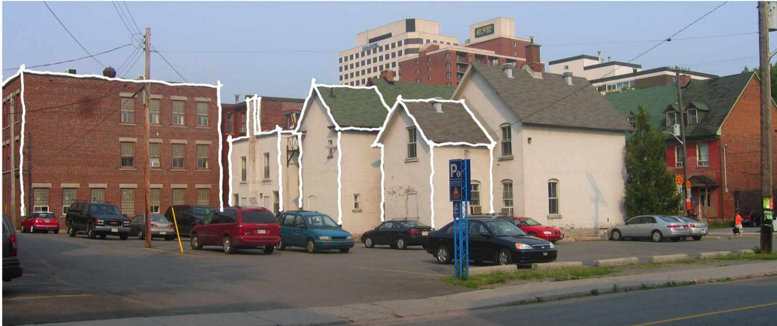
VIEW FROM CUMBERLAND STREET SHOWING REAR ADDITIONS TO BE DEMOLISHED
