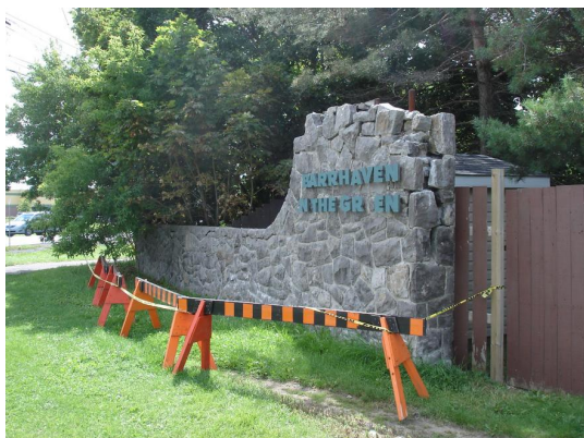
Example of gateway feature without proper construction techniques to protect stone from moisture. City of Ottawa, Greenbank and Wessex.
