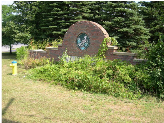
Problems with painted wood sign, no coping to protect brick wall, unruly plant material and lack of maintenance. City of Ottawa, Wyldewood Subdivision
