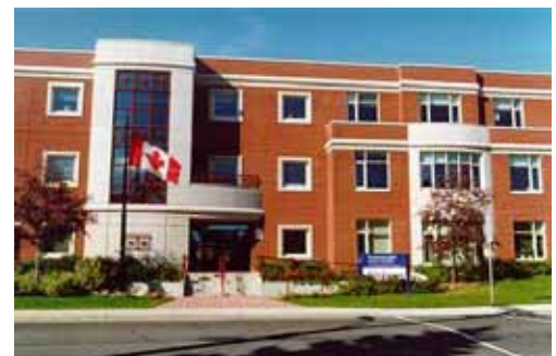
To this: Multi-storey schools close to the street, easier to walk to, with open space that doubles as a public park.
