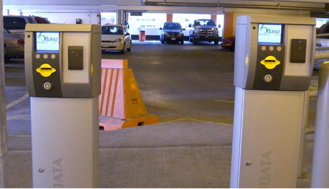
New Skidata entrance terminals in the ByWard Market parking facility at 70 Clarence St.
