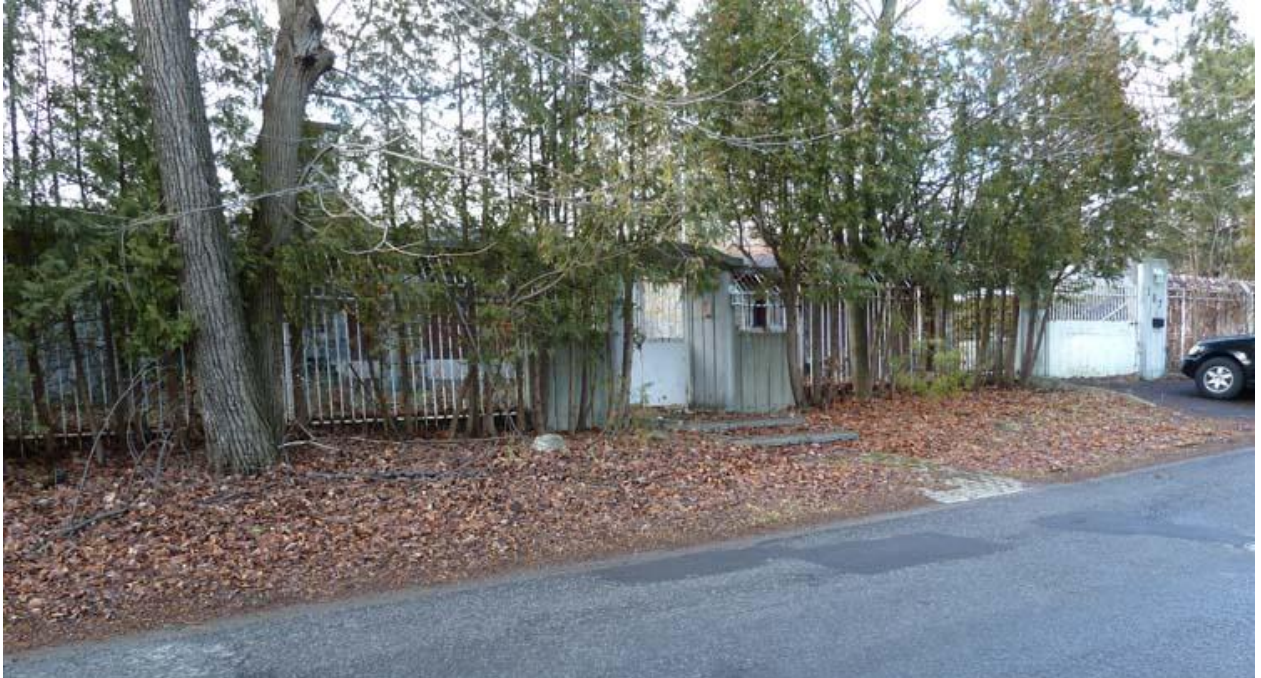
Figure 9: View of the front fence and gate erected in 1979. (Contentworks Inc., 2011)
