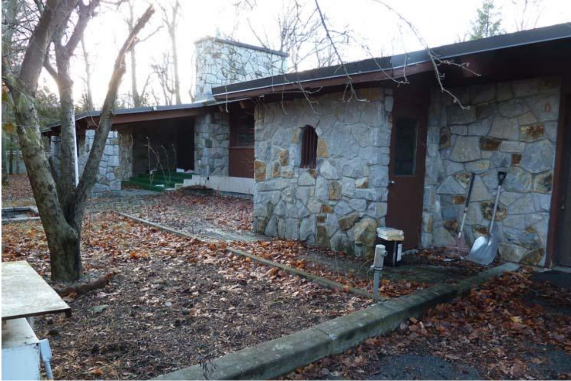
Figure 7: Front elevation of 187 Lansdowne Road. The projection with the rounded window was added in 1979 as part of the remodeling of the garage. (Contentworks Inc., 2011)
