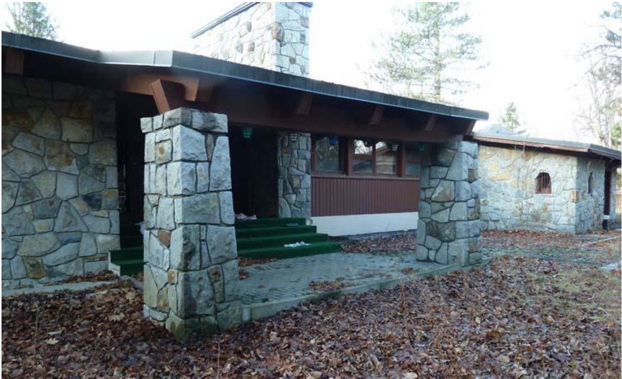
Figure 8: Front entrance of 187 Lansdowne Road, with guardhouse and garage visible on the far right. (Contentworks Inc., 2011)
