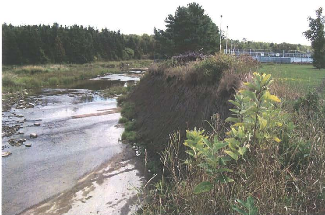
Photo No. 1: Critical slope surface (east side)
