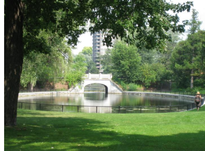
FIGURE 26: PATTERSON CREEK AND O'CONNOR STREET BRIDGE
