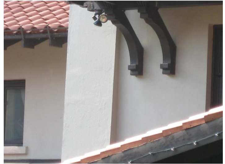
FIGURE 30: SMOOTH STUCCO CLADDING AT 85 GLEBE AVENUE
