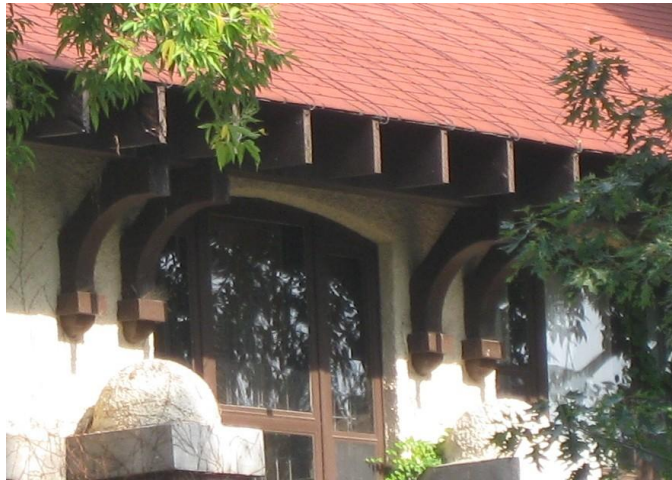
FIGURE 36: WOOD EAVES BRACKETS
