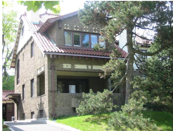
FIGURE 34: PORCH ON CLEMOW AVENUE
