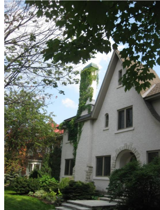
FIGURE 38: CATEGORY 2 BUILDING AT 38 MONKLAND AVENUE
