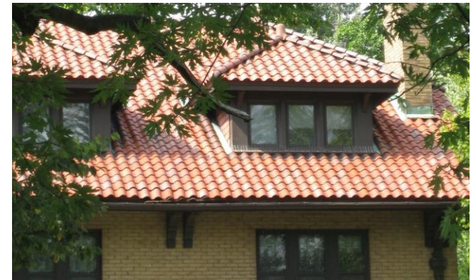
FIGURE 29: CLAY TILE ROOF
