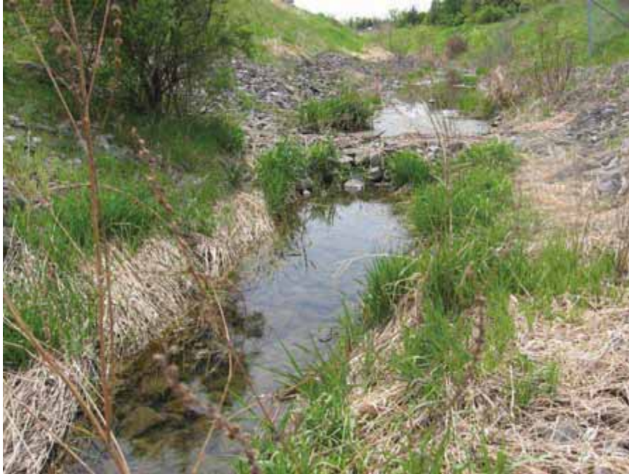
Figure 25. Photograph taken looking upstream through potential ROW (all corridors) at rock check dam and general bank vegetation.
