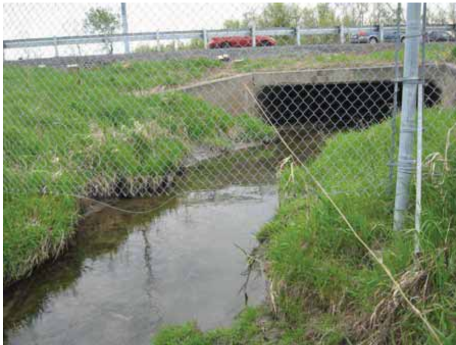
Figure 10. Photograph taken looking upstream at Highway 417 culvert for Tributary A and the general channel characteristics of this watercourse.
