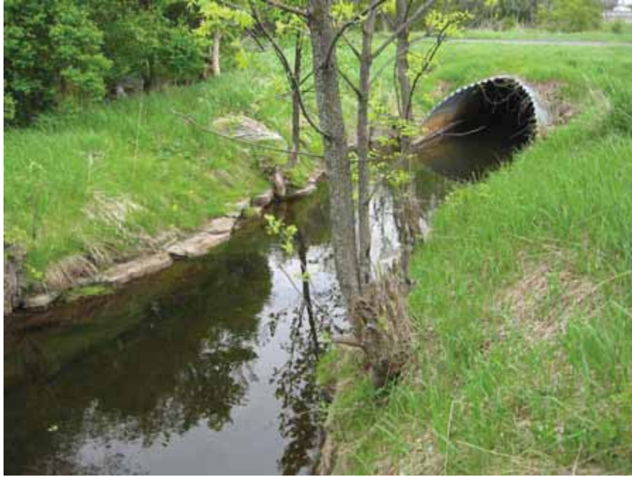
Figure 9. Photograph taken looking downstream at inlet of culvert at recreational trail.
