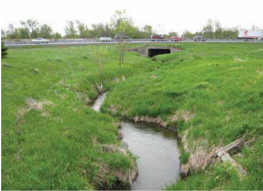
Figure 1. Photograph taken looking upstream at general channel characteristics between Highway 417 ROW and Corkstown Road.
