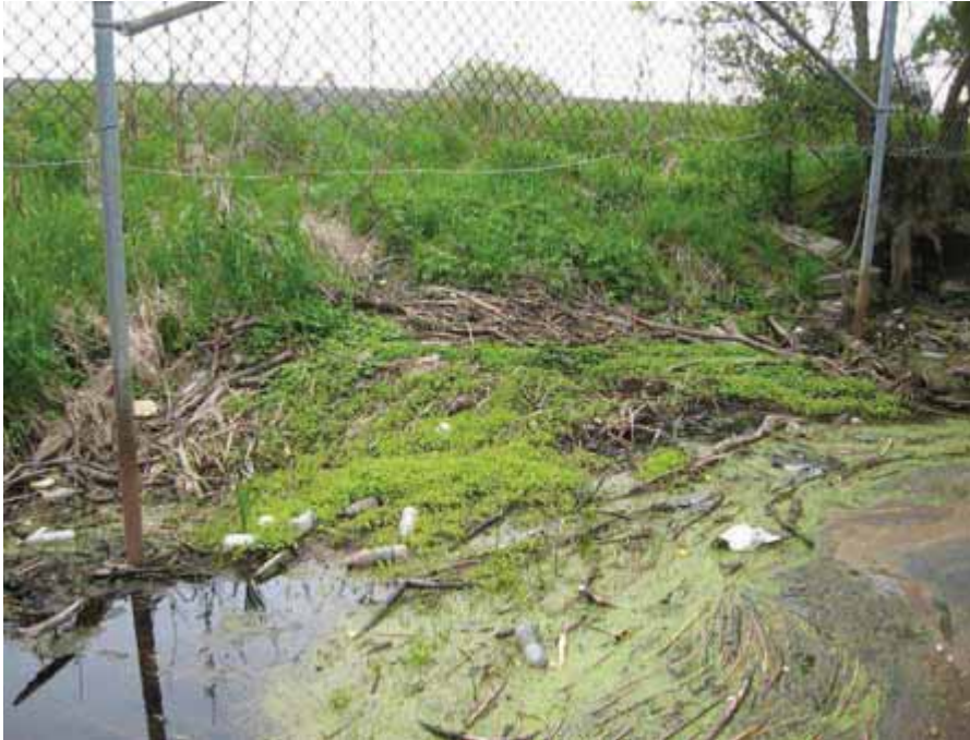
Figure 5. Photograph taken looking downstream at the general location of Corkstown Road crossing, and the debris burying the inlet.
