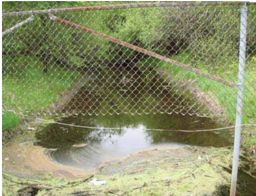
Figure 4. Photograph taken looking upstream from Corkstown Road at general characteristics of Stillwater Creek upstream of road crossing.
