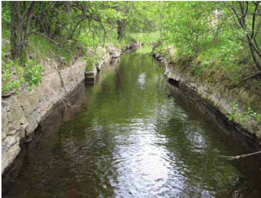
Figure 8. Photograph taken looking downstream at general channel characteristics of Stillwater Creek where it is confined within the bedrock walls, between Corkstown Road and the recreational trail.
