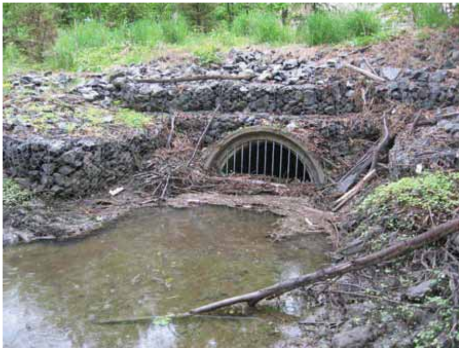
Figure 20. Photograph taken looking downstream at the culvert leading into the storm sewers and the woody debris accumulation on banks and in front of the grated culvert.
