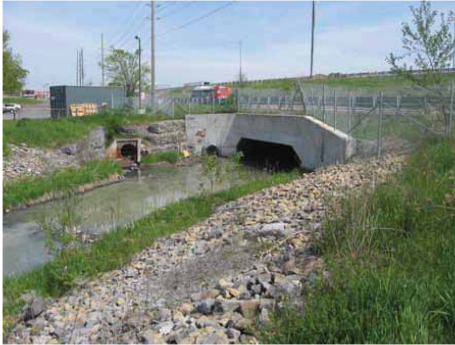
Figure 27. Photograph taken looking upstream at the bridge over Graham Creek for Highway 417.
