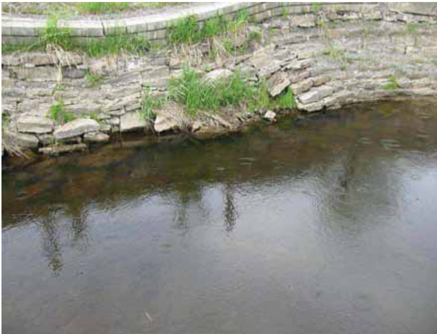
Figure 6. Photograph taken looking upstream at the outlet of the Corkstown Road crossing and failing retaining wall.
