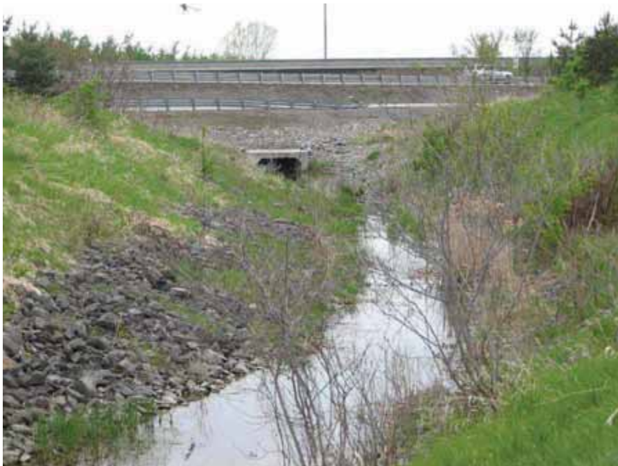
Figure 24. Photograph taken looking upstream at the culvert under Highway 417 for this tributary.
