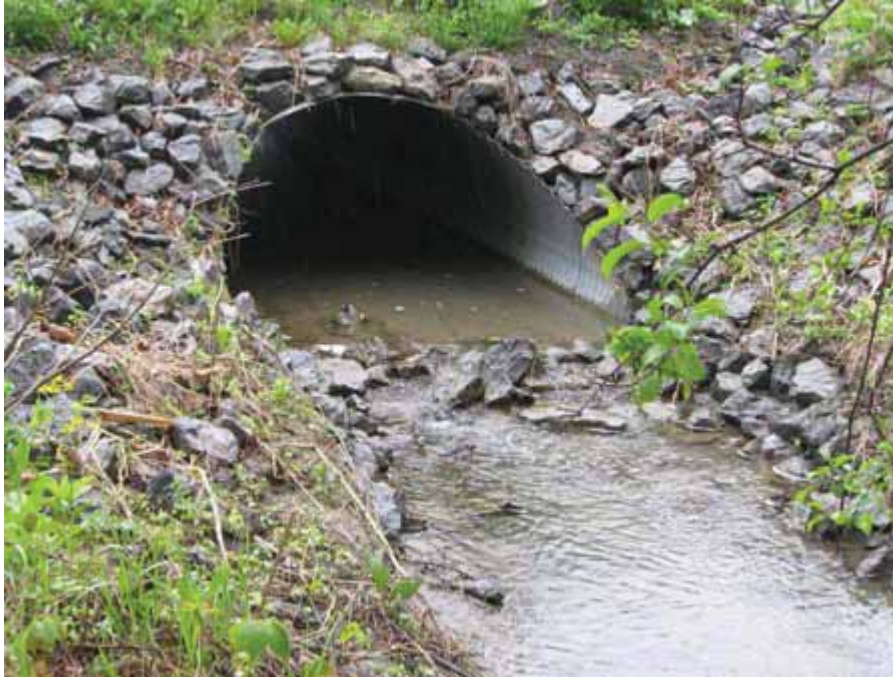
Figure 17. Photograph looking upstream at the culvert installed at the recreational trail and the rip rap bank protection and rocky ramp.
