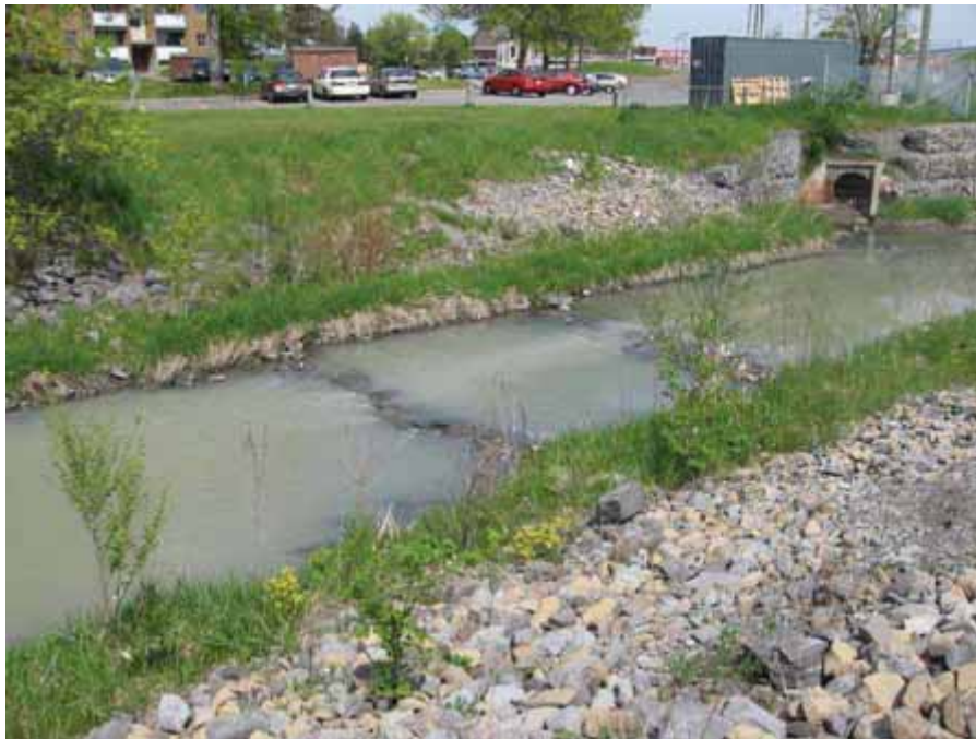
Figure 28. Photograph taken looking across channel from western bank at the manmade riffle features and turbid (grey-water) observed during the 2009 field investigation.
