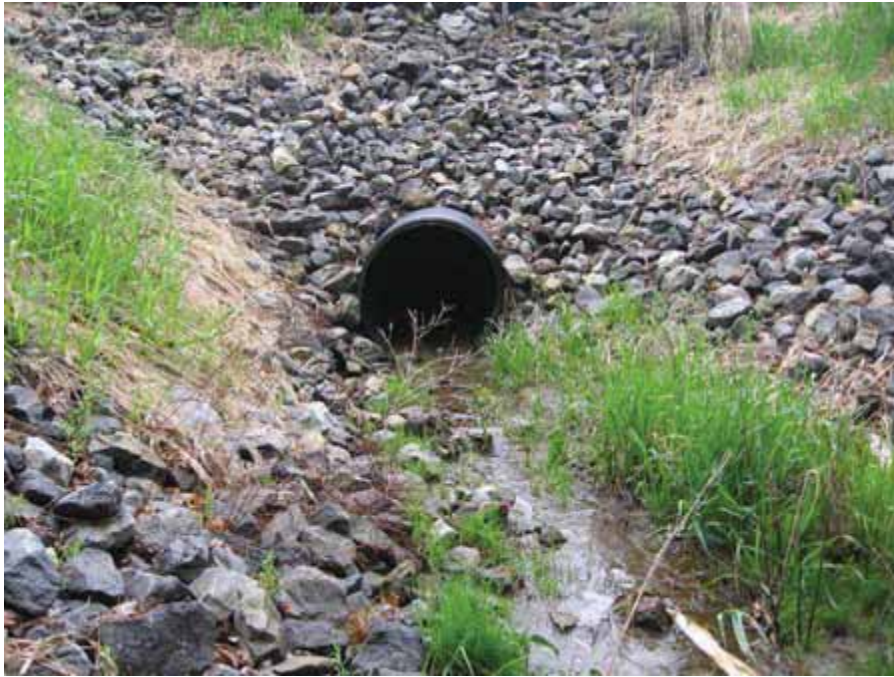
Figure 13. Photograph taken looking upstream at the culvert under Highway 417 for this tributary.
