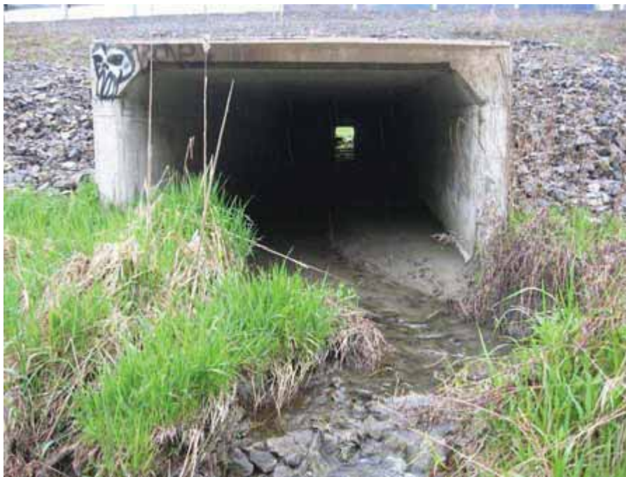
Figure 16. Photograph taken looking upstream at the box culvert for this tributary under Highway 417.
