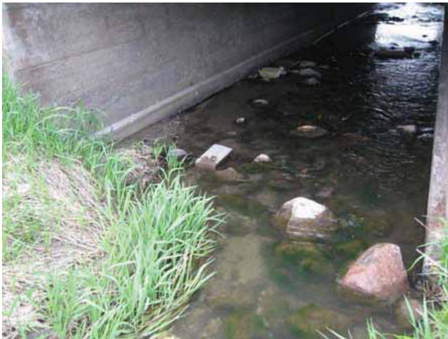
Figure 2. Photograph taken looking downstream at the Corkstown Road culvert and the substrate.
