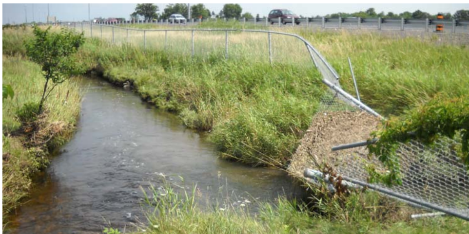
Figure 3-1: On-going Erosion of Stillwater Creek at C3
