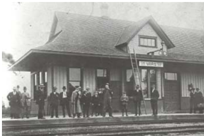
Vars railroad station
