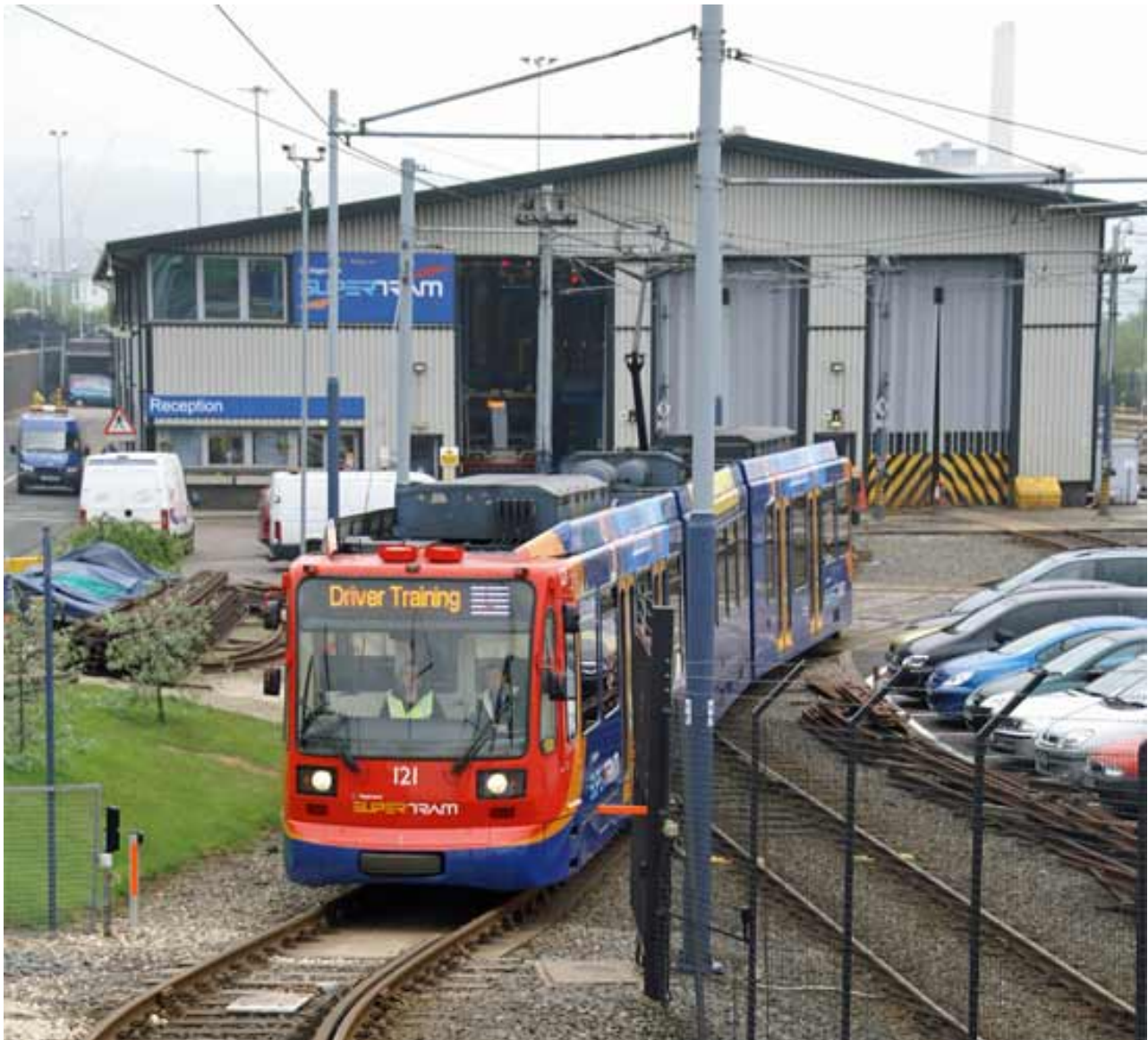
The Sheffield Supertram maintenance facility (same fleet size as OLRT). (This scale of facility will serve as the NLRT heavy maintenance centre)
