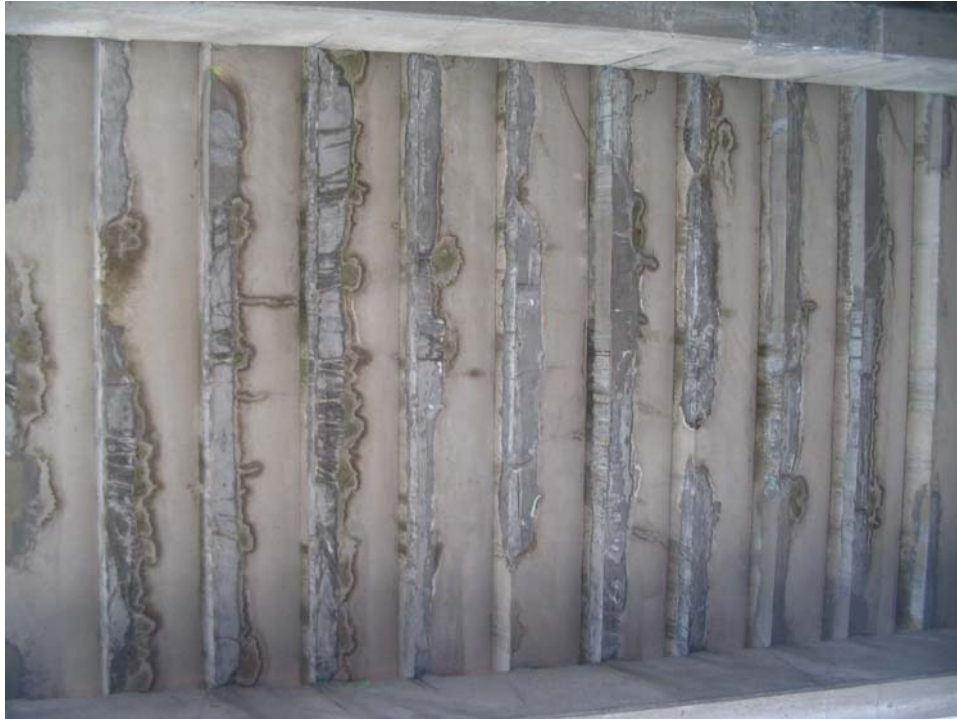
Photo 09 – Precast Seating Panels: typical soffit repair patches
