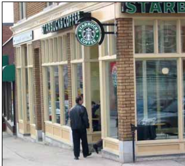
Figure 19: Compact signs fit in with the design of the building.
