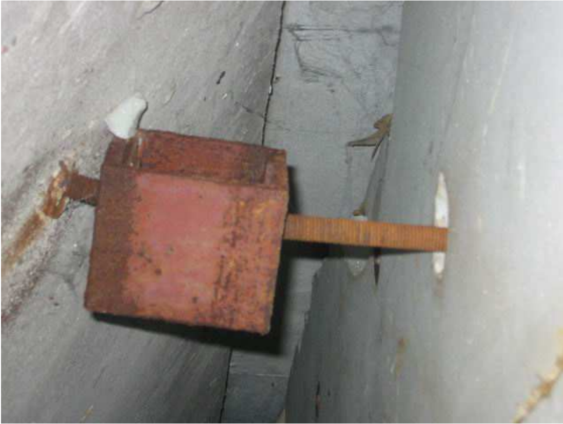
Photograph 21 - Anchor for angled panel
