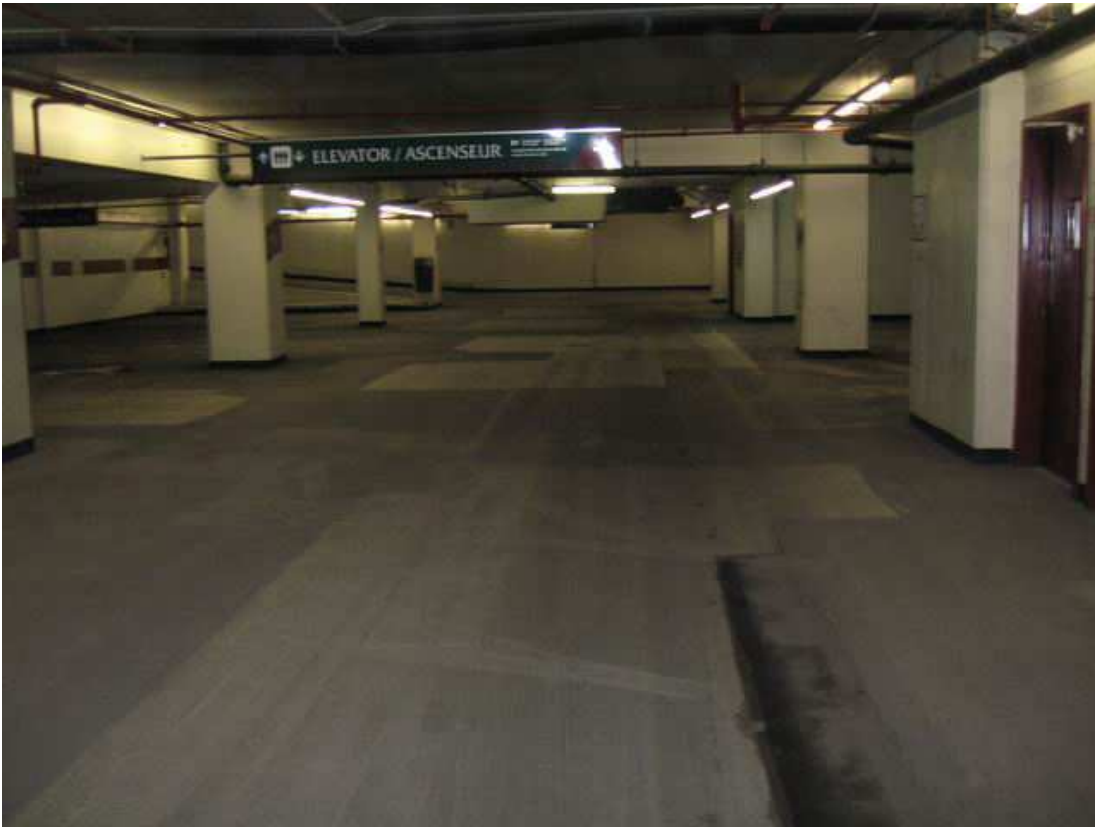
Photograph 7 - Membrane patch repairs
