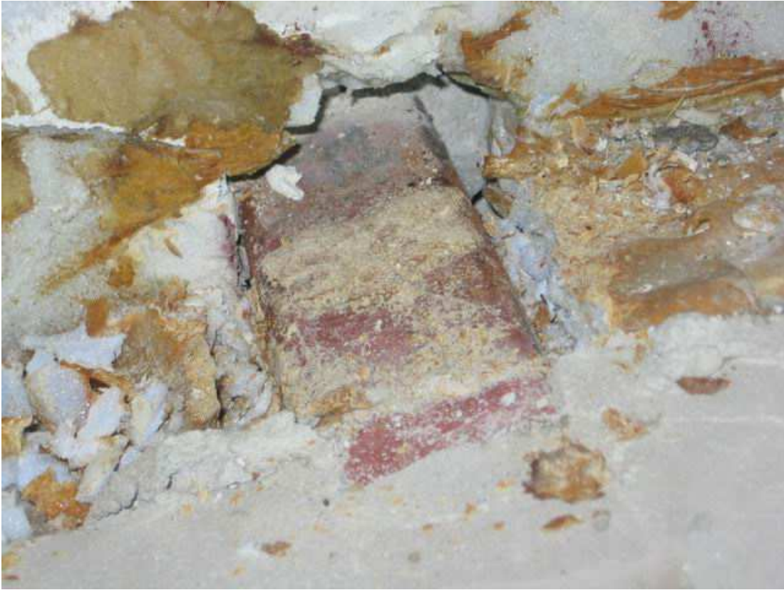
Photograph 19 - Panel connection at floor slab
