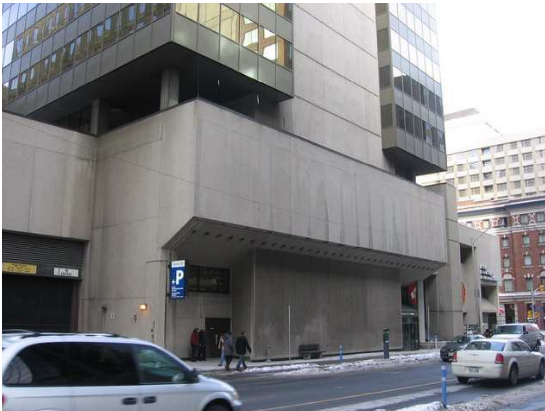
Photograph 2 - Laurier Avenue Elevation
