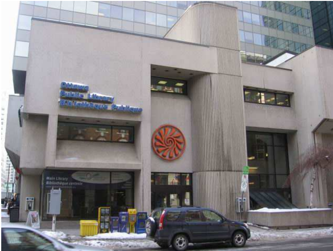
Photograph 1 - Metcalfe Street elevation
