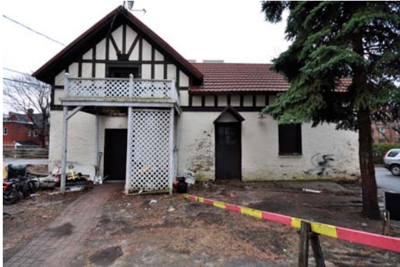
1 1/2 storey garage looking South
