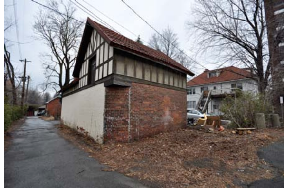
Rear of garage showing laneway looking West
