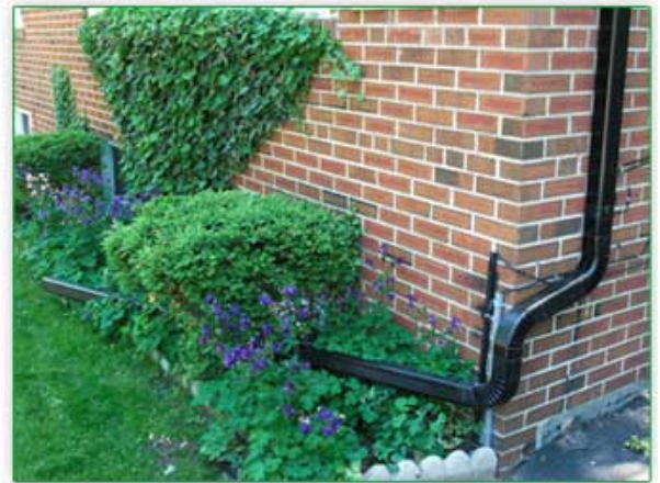
Figures 1a and 1b Downspout Redirection 6
