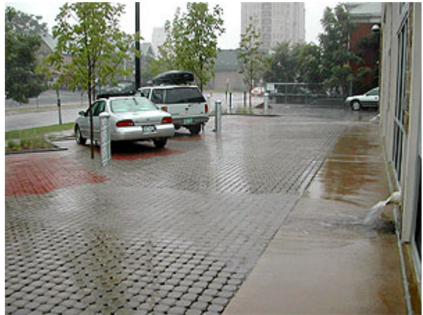
Figure 5a: Porous Pavers used for a Walkway and Parking Area 11
