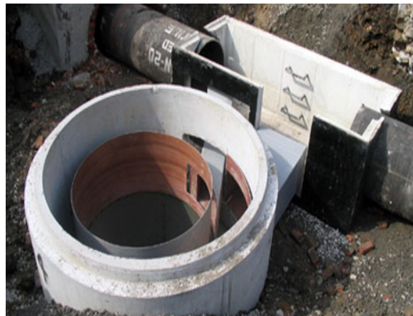
Figure 11b: Typical Installation of a CDS Unit 22
