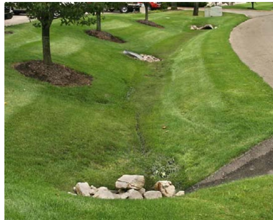
Figure 6a: Roadside Grass Swale 13
