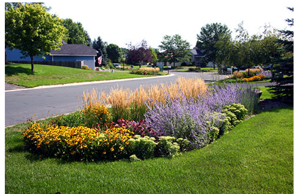
Figure 4b: Rain Garden 10
