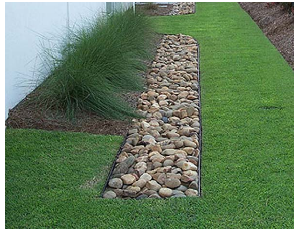
Figure 7: Side Yard Infiltration Trench 15
