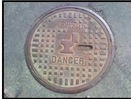
Figure 8 – Maintenance Hole Cover Replacement
