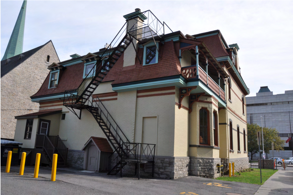
GRANT HOUSE SHOWING EXISTING CONDITIONS
