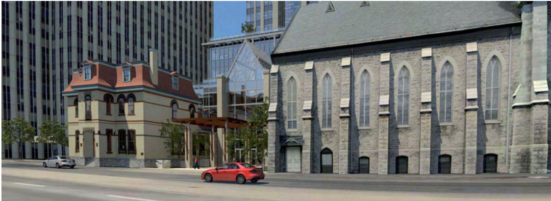
VIEW FROM ELGIN STREET SHOWING PARKETTE AND ENTRANCE TO WINTER GARDEN
