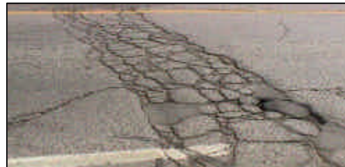
UTILITY TRENCHING DAMAGES ROADS
