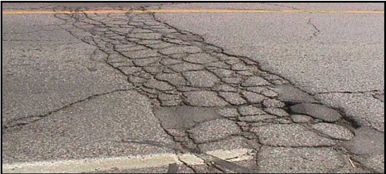
Figure 6: Utility trenching permanently damages roads
