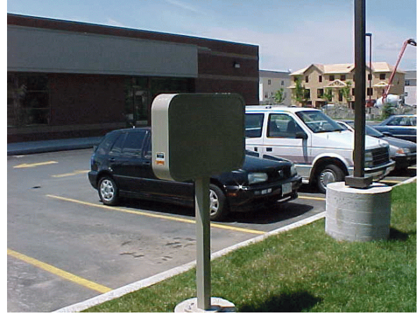
Opaque backing on Directional Sign
