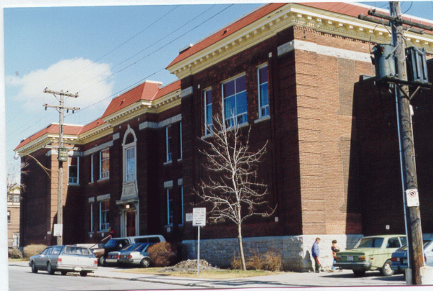
North (rear) facade, constructed 1920 (City of Ottawa Heritage Section)
