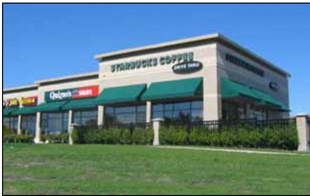
Figure 19: The low wall along the edge of the site screens the driveway from view.
