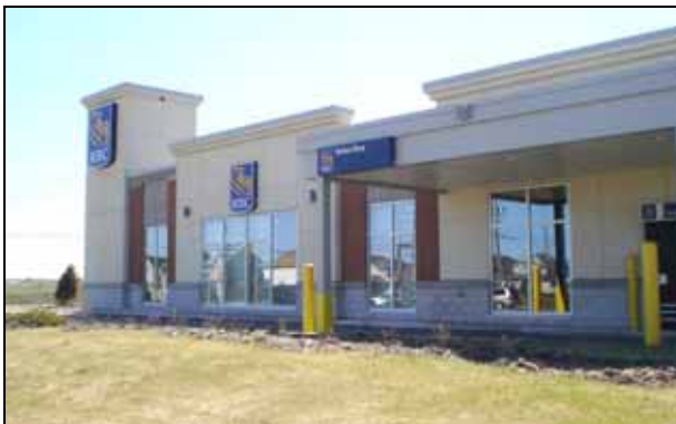
Figure 5: Employee rooms with glass windows are located facing the public areas in this drive- through bank.
