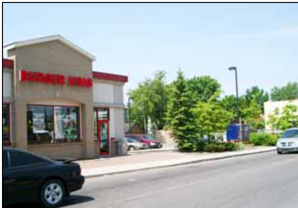
Figure 7: This drive-through restaurant has a customer entrance directly accessible from both the public sidewalk and the parking area.
