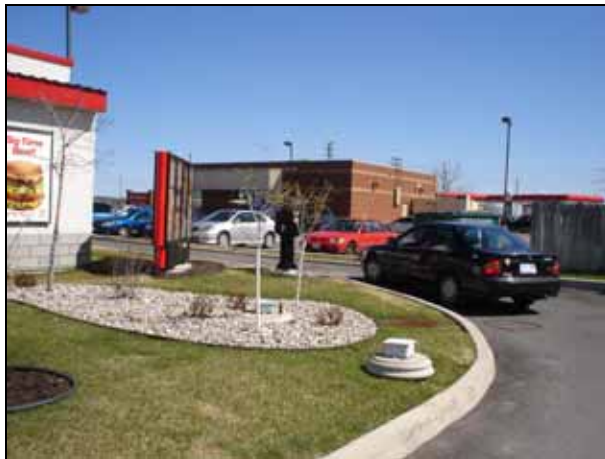
Figure 21: The planting area collects and stores stormwater.
